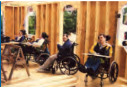
Skills' "foremen" regularly checked progress on the construction of their new home.
